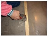
Staple plastic to wood. This will hold the plastic in place while you wrap the plastic, one turn around the wood.
