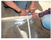
Cut a 2 - 4 ft by 4 ft pieces of plastic. One for each end. Now get a 1 in by 2 in by 4 ft piece of fir and staple the plastic to the bottom of the 4 ft piece of plastic. It will take about 5 staples to secure the plastic. This will hold the plastic in place while you roll it under one turn.
