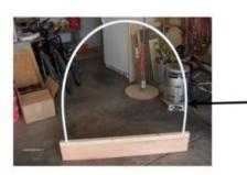
Cut end PVC 109 inches (it is slightly shorter than the standard 10 ft pieces that will be used for the 3 middle hoops).
