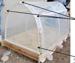
1 in by 2 inch by 4 inch blocks, screwed through plastic and attached to 1 in by 2 in by 8 ft purlins
