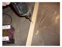
Now place a 1 in by 2 in by 8 ft fir on top of 2 in by 2 in by 8 ft fir and screw in using 1 5/8 in screws (use 5 screws per side).
