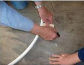
In the bottom picture note that we are wrapping the plastic around the PVC. Every 12 inches or so we are poking a hole in the plastic as close to the PVC pipe as we can get. This hole is to fit a 4 inch or 6 inch cable tie through the hole and it is pulled tight.
