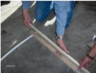
Now using 1 7/8 inch screws secure the 1 in by 2 in by 4 ft
