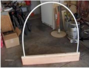
Cut end PVC 109 inches (it is slightly shorter than the standard 10 ft pieces that will be used for the 3 middle hoops).
