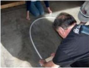
It is now time to cut the plastic to fit the end hoop. Note in picture #2 that someone needs to hold the plastic sheet tight while someone traces around the hoop.
