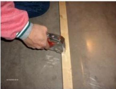
Staple plastic to wood. This will hold the plastic in place while you wrap the plastic, one turn around the wood.
