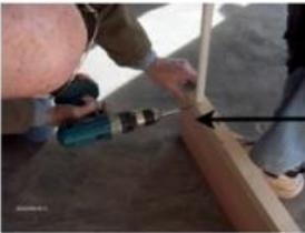
Secure PVC to end using a 1 1/4 inch screw
