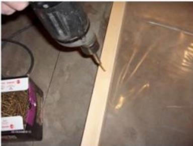
Now place a 1 in by 2 in by 8 ft fir on top of 2 in by 2 in by 8 ft fir and screw in using 1 5/8 in screws (use 5 screws per side).
