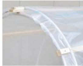
10 ft 1/2 inch PVC cut to fit under end hoop (about 9 ft but you will need to measure to be sure).
